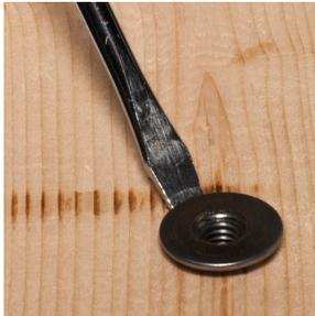
Remove the old metal insert with a screwdriver.
