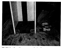
7) Slide the three-panel shaft unit over the blocking, then attach. Apply glue to exposed vertical edges of panels.
