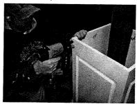
8) Attach final panel. For use as a newel, additional blocking should be added between panels and post (post would be cut off at height of shaft.)
