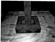
1) Install blocking around load bearing support (typically pressure treated post). Blocking should be made from pressure treated wood, and must be the same size as the inside of the pedestal/newel.
