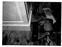
9) Apply glue to backs and mitered edges of base moldings, then assemble to bottom of platform (same as no-taper column bases).
