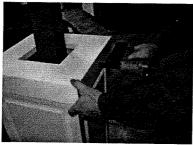
11) Apply glue to backs and mitered edges of cap moldings, then assemble to shaft below top platform with screws or pin-nails.
