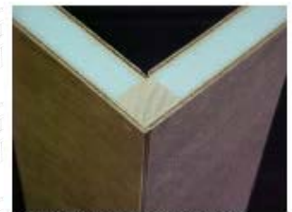
Inside Corner Post Joint
